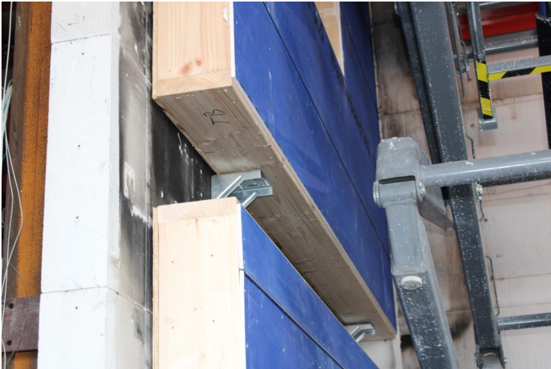
Photo No. 1 Prefabricated cassettes being mounted.
