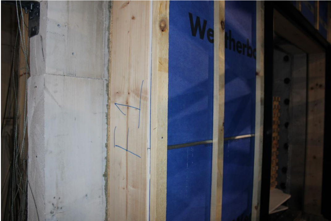
Photo No. 5 Vertical formworks have been mounted.
