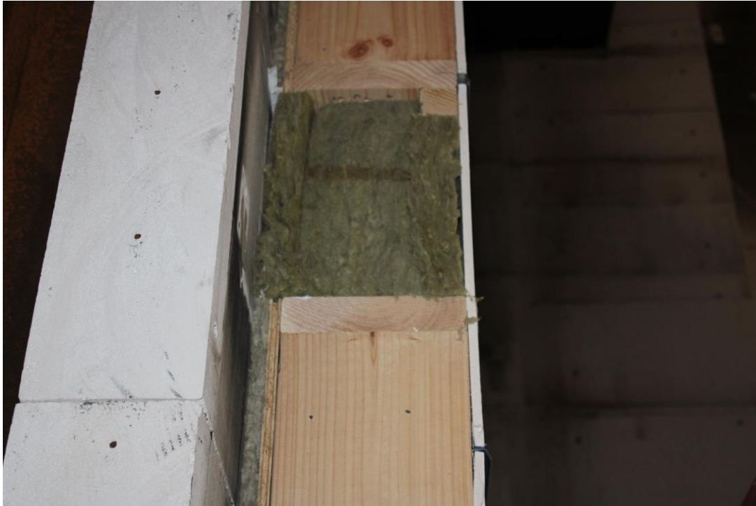
Photo No. 3 Insulation in the gap between two cassettes.
