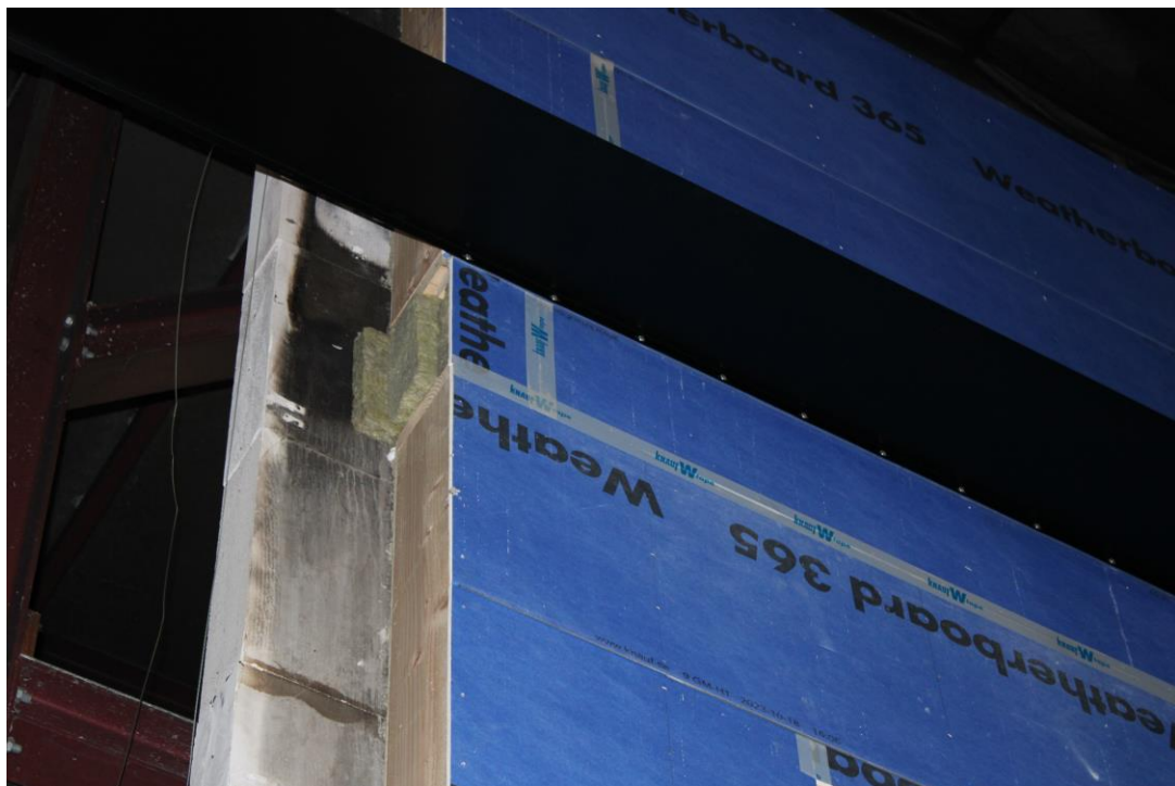
Photo No. 4 Flame deflector is being mounted.
