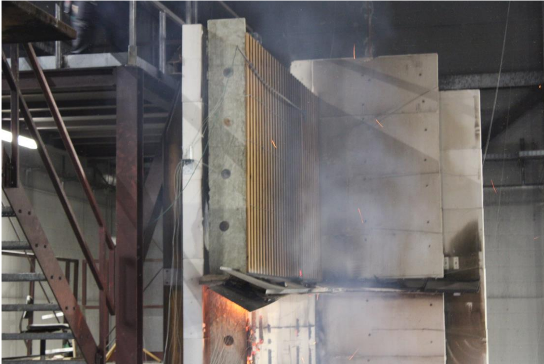
Photo No. 21 Ember from second floor 43 minutes into the test.
