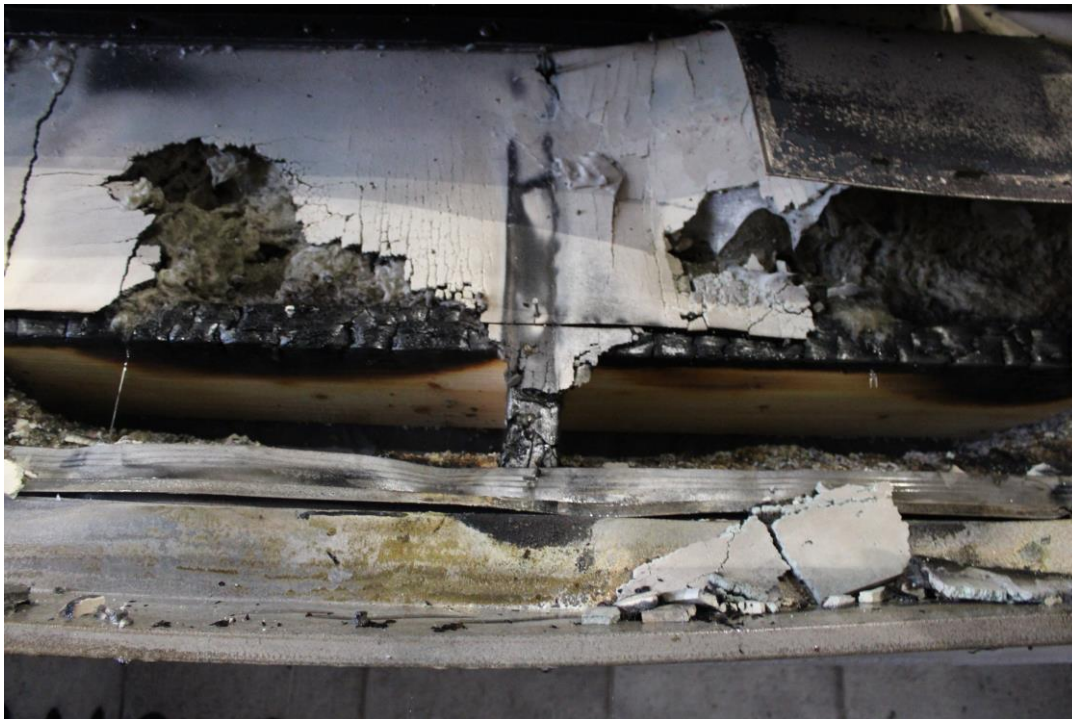
Photo No. 24 Test specimen after the test. Detailed photo of the top of fire chamber.
